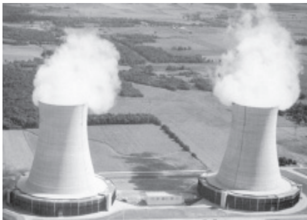
Plant Vogtle in Waynesboro is a Nuclear Power Plant in Georgia.
